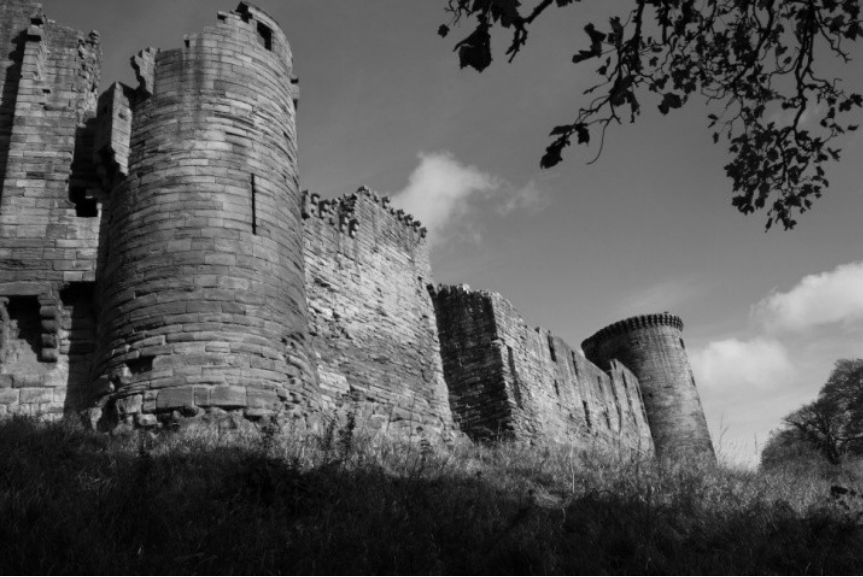
Bothwell Castle - the south curtain wall – Photograph by Ian Beckett
