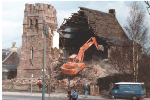
Demolition of Kirkfield Church
