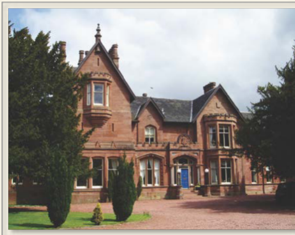
Elmwood House today
